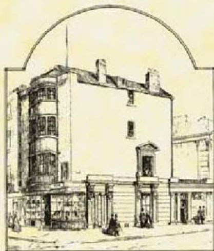
'The 1789 premises at 219 High Street Exeter'
